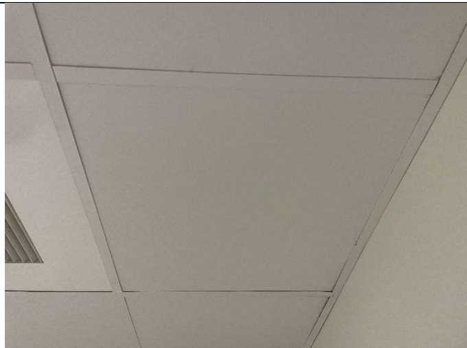
Photo 29: HM-BB: 2' x 2' Drywall Ceiling Tile, White
