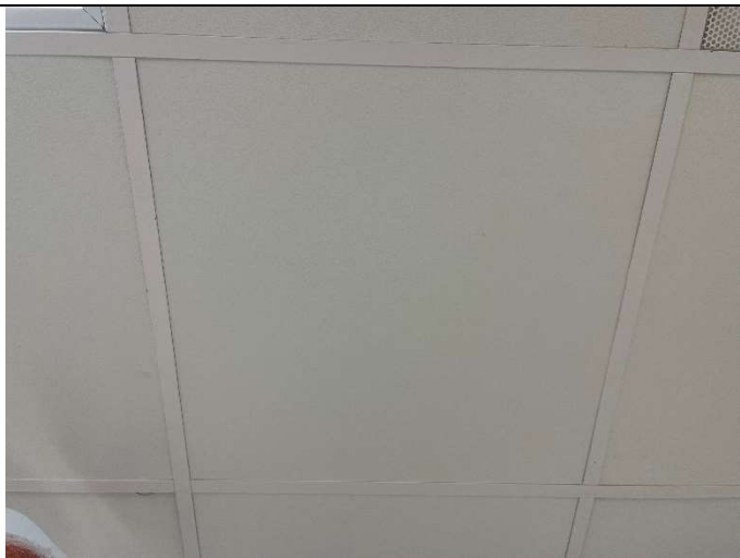
Photo 17: HM-P: 2' x 2' Drywall Ceiling Tile, White
